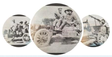
The Model T Ford was one of the most widely recognised vehicles of its time. Mass produced in both the US and UK, it was ruggedly constructed, simple
